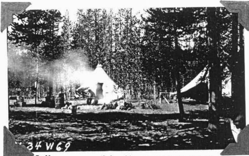
Spike camp used by the enrollees in the construction of Bear Creek Snowshoe Cabin. September 11th, 1934
