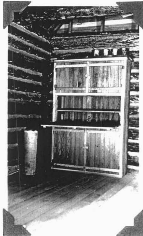
Cabinet installed in cabin September 4th, 1934
