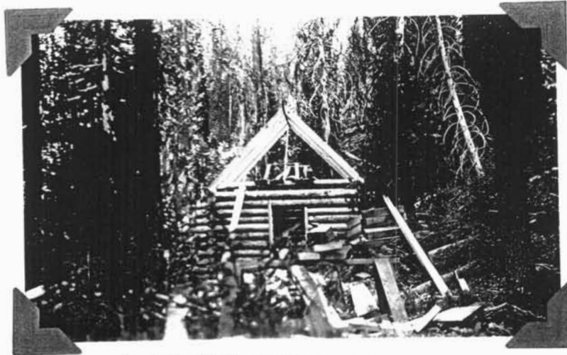
Front view, roof framing in place September 29th, 1934
