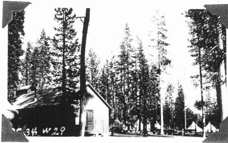
Messhall and Enrollees' quarters Camp Oregon Caves, built with CCC Enrollees from this Camp Oregon Caves Project No. September 8th, 1934
