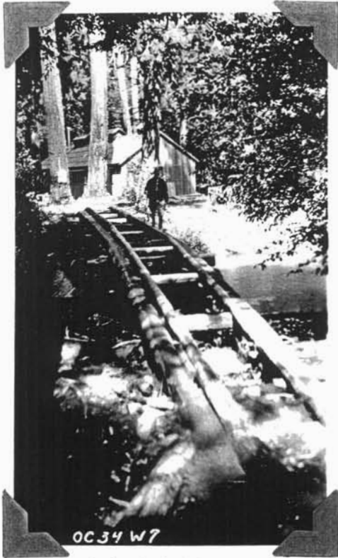
Original Bridge over Sucker Creek June 1st, 1934
