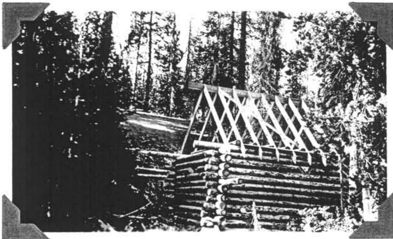
Rear view of roof framing in place September 29th, 1934
