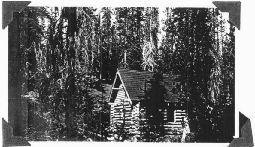
Cabin nearly complete, rear view October 6th, 1934
