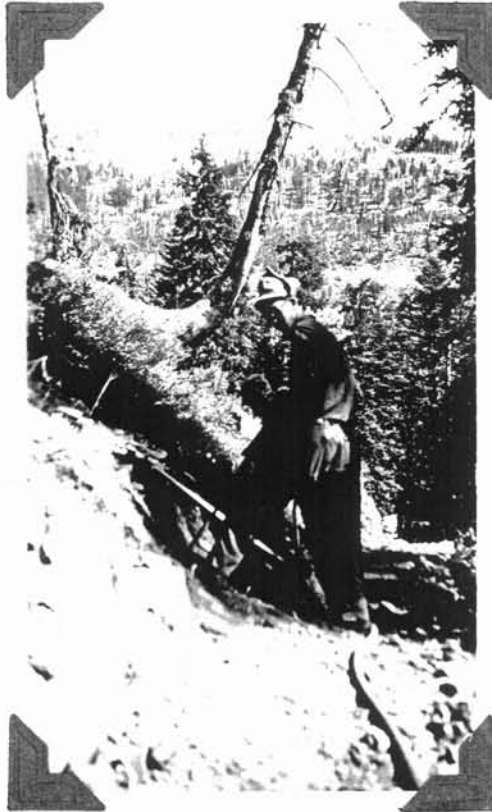
Enrollee using Air Jack Hammer in Construction of Trail September 24th, 1934
