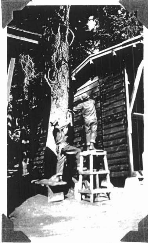
Painting Lumber Sheds with spray gun October 3rd, 1934
