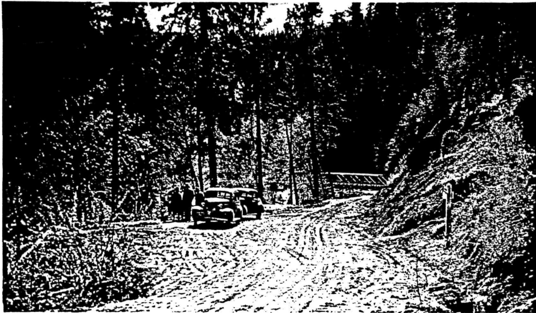
Bridge across South Fork of Coquille River Forest Service Road, within Squaw Basin (#12) Area. Foot of trail to Squaw Creek etc.
